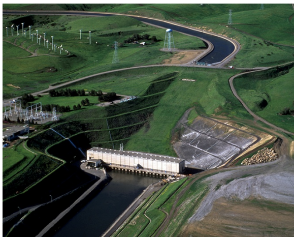
Harvey O. Banks Pumping Plant.
