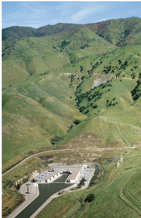
A. D. Edmonston Pumping Plant.
